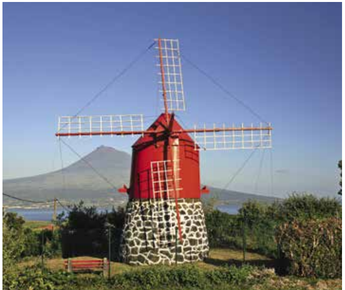
Espalamaca Windmills (19 th /20 th centuries) - These windmills have two floors, with the Portuguese influence being visible in the eight poles where the triangular sails are tied. The Flemish have also influenced their design, namely in the square grids of the sails. Some of these windmills have been classified for their architectural and historic interest.
